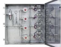
Complete custom panel solutions incorporating best-in-class fluid contol & pneumatics products with PLC and electrical components. An optimized, engineered solution for your pilot valve control and other pneumatic automation needs.
