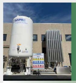
Independent LNG facilities for faster high pressure and cryogenic testing also on large sizes ball valves, high pressure up to 1000 bar for very special applications. Qualified personnel to carry out specific testing according to customized procedures.
